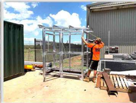
Measuring the new toilets
